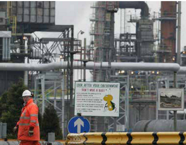
Disruptions to national fuel supplies would greatly impact the economy
